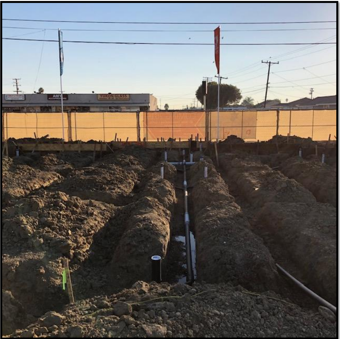
Ground plumbing installed building 1
