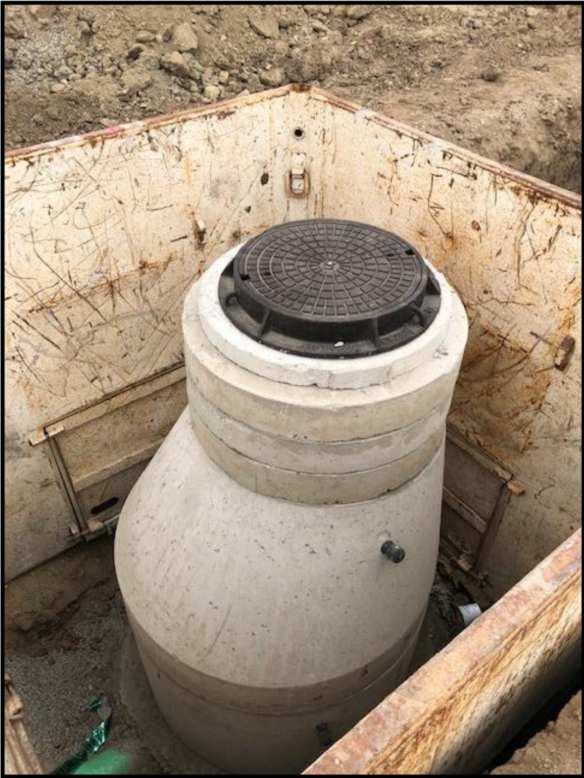
Sewer manhole stacked 1
