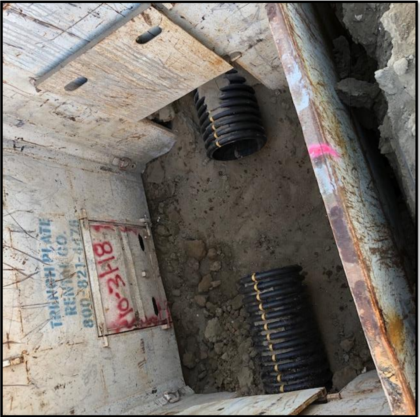
Storm drain manhole being prepped
