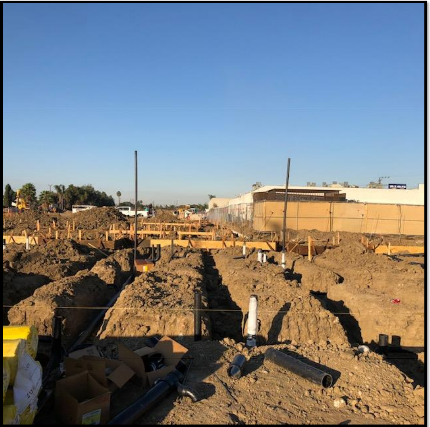
Ground plumbing installed building 2
